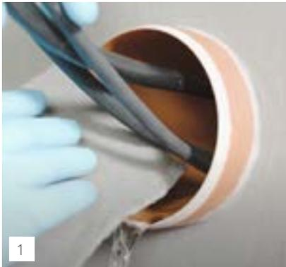
1 The application area flanks must be thoroughly cleaned with an abrasive pad and with KÖSTER Cleaning Brush from the inside so that they are free of dust, sand and other loose particles.
