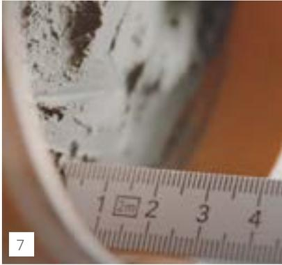
The sealing compound is recessed 1-5 cm (depending on cable thickness and weight) from the wall surface and smoothed with KÖSTER Spatula.
