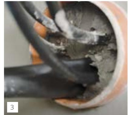
Finally, the penetration is resealed by pressing additional KÖSTER KB-Flex 200 around the cables.
