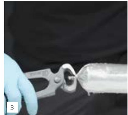
3 Remove the KÖSTER KB-Flex 200 tubular bag from the warm water (maximum +40 °C) and cut off the front clip of the tubular bag.
