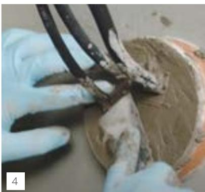
As an additional safeguard and to hold the pipe/cable centered, the exposed material is covered again with KÖSTER KB-Fix 5.
