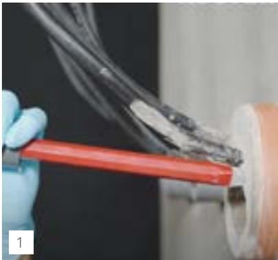
If a new cable is to be installed in this penetration later on, the KÖSTER KB-Fix 5 plug is first removed with a hammer and chisel.
