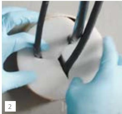
2 Before applying KÖSTER KB-Flex 200, a backing is installed in the penetration at a depth corresponding to the installation depth (consult Technical Data Sheet) using e.g. a common PU foam.
