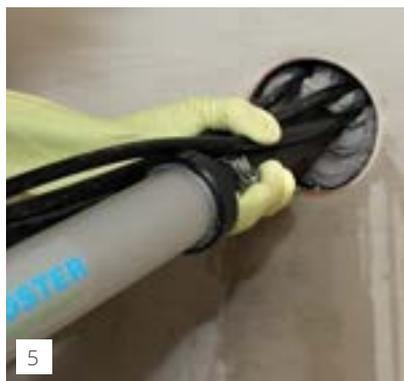
5 The KÖSTER KB-Flex 200 material is pressed into the penetration from back to front. Waterproofing made of KÖSTER KB-Flex 200 must be dimensioned so that the ratio of the depth (d) to the width (w) of the installed material is not below 1.5:1. The minimum depth should not be below 8 cm. The maximum diameter of the waterproofing is 300 mm.
