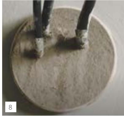
As an additional safeguard and to hold the pipe/cable centered, the exposed material is covered with KÖSTER KB-Fix 5.
