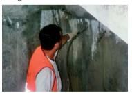
Injection using a low pressure system
